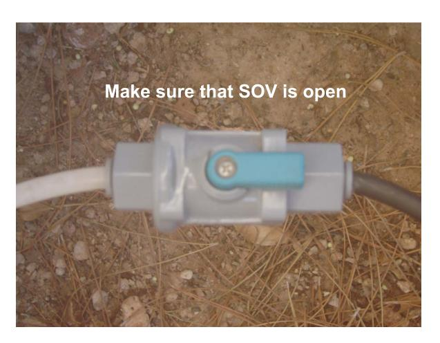
If you do not want to use the by-pass fitting, you can simply reroute the tubing through one shut-off valve.
