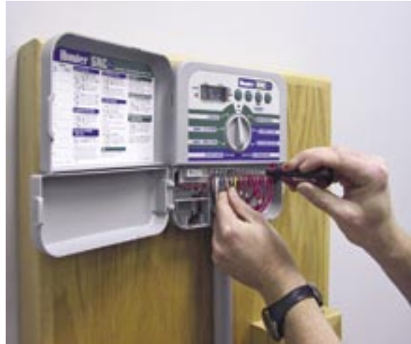
Use color-coded irrigation wire to connect the valves to the controller. You will need one wire for each valve, plus one common wire.
