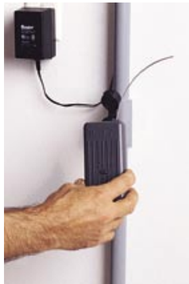
Use color-coded irrigation wire to connect the valves to the controller. You will need one wire for each valve, plus one common wire.
